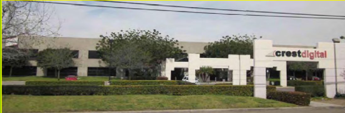
3845 Coronado Street 109,000 Square Feet Leased!
