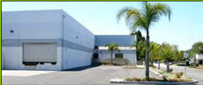
1220 Kona Drive 24,325 Square Feet Leased!
