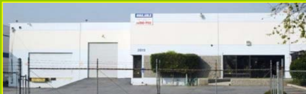
2019 Acacia Court 14,168 sq ft of Warehouse Leased!
